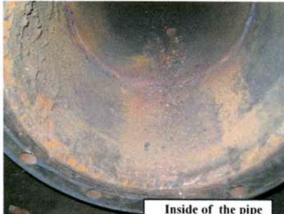
Inside of the pipe
