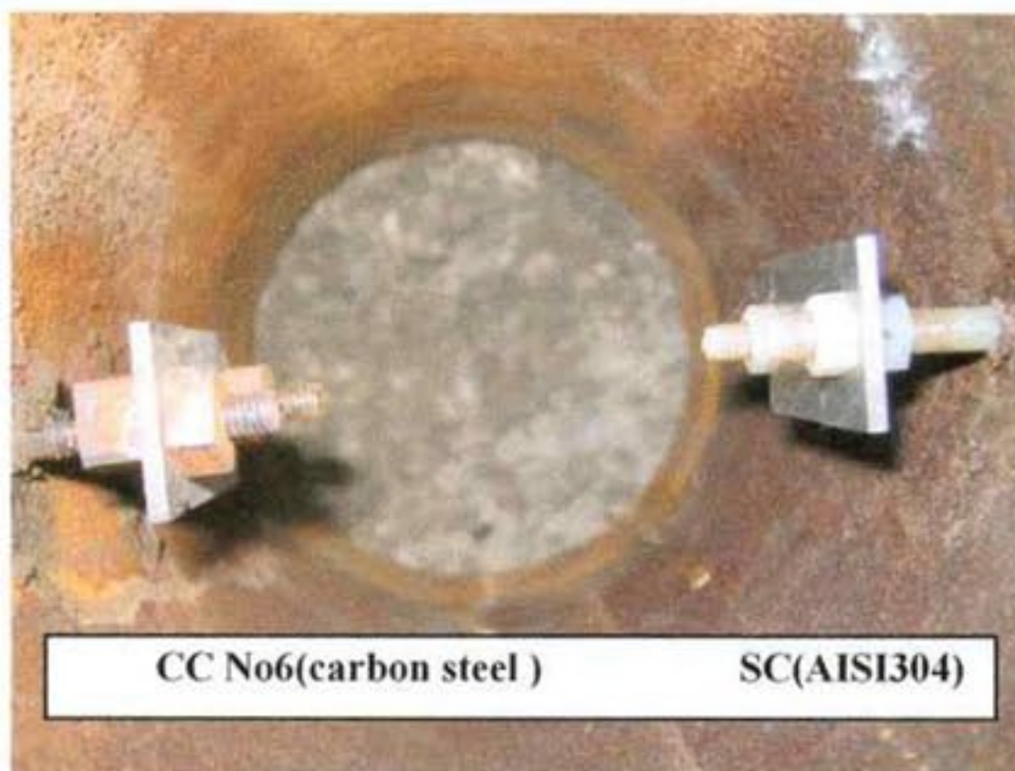
Fig.(5): Shows the installation of the Corrosion Coupon and Scale Coupon in Position No. 2(4 inch)
