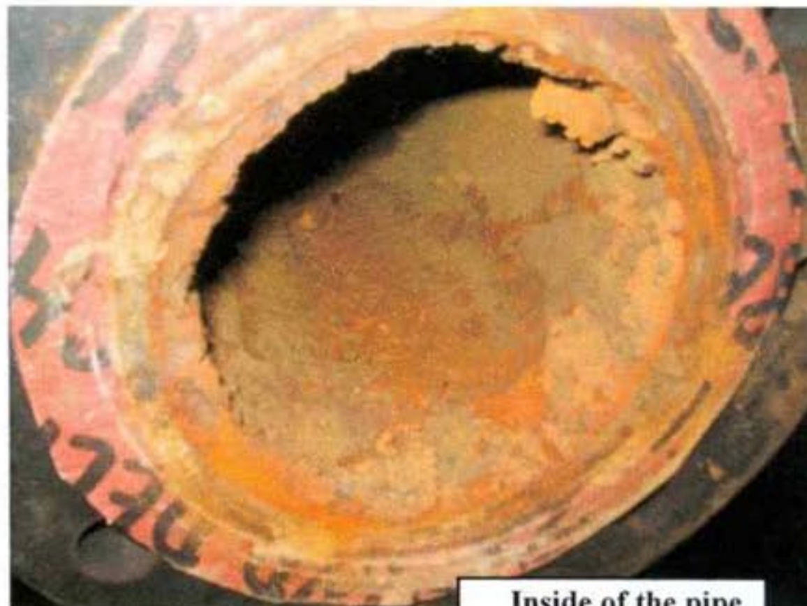
Inside of the pipe
