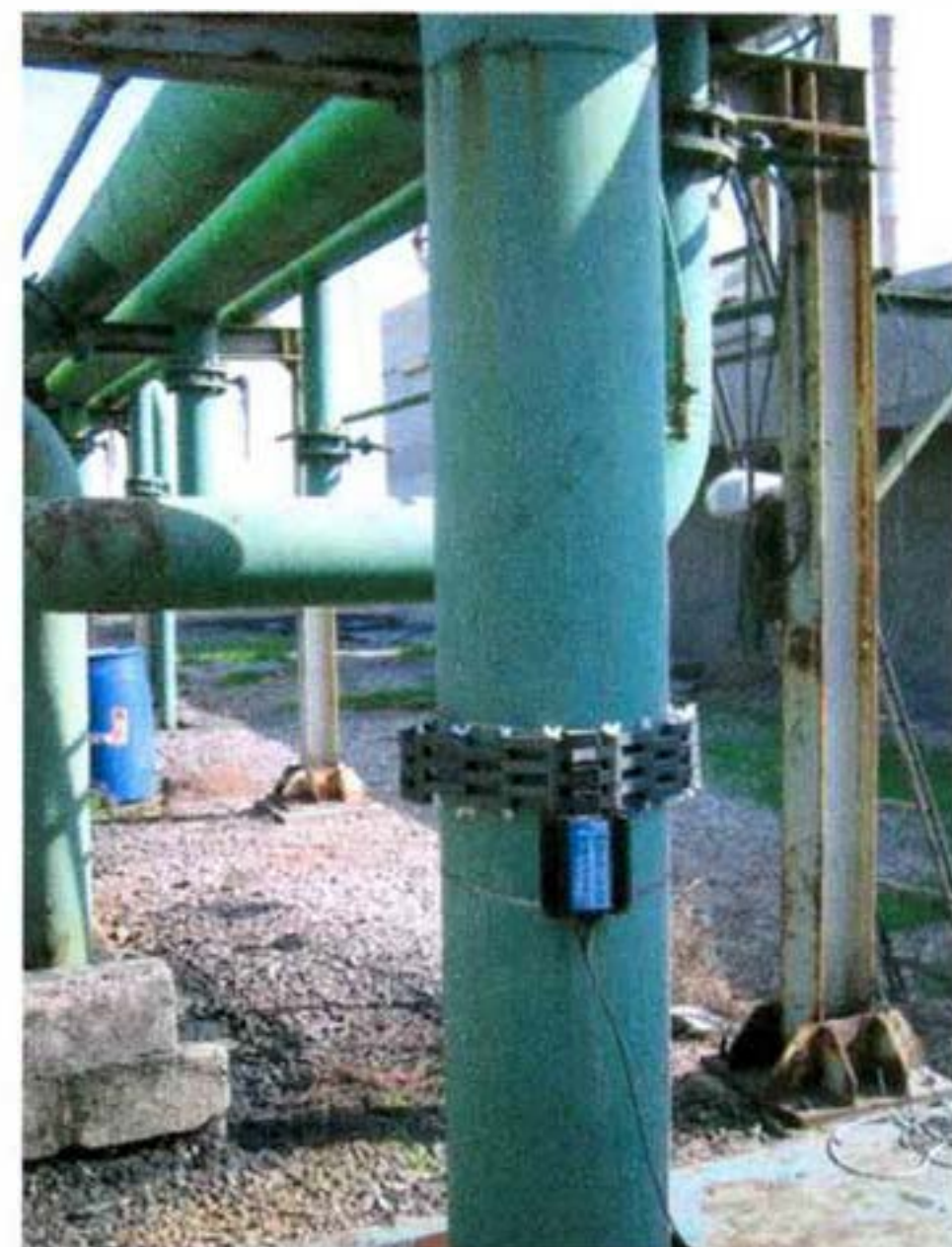
Fig.(1) Hydroflow technology ( photo to the left) connected to one of the pipes in a selected location of JORDAN STEEL FACTORY ( photo to the right).
