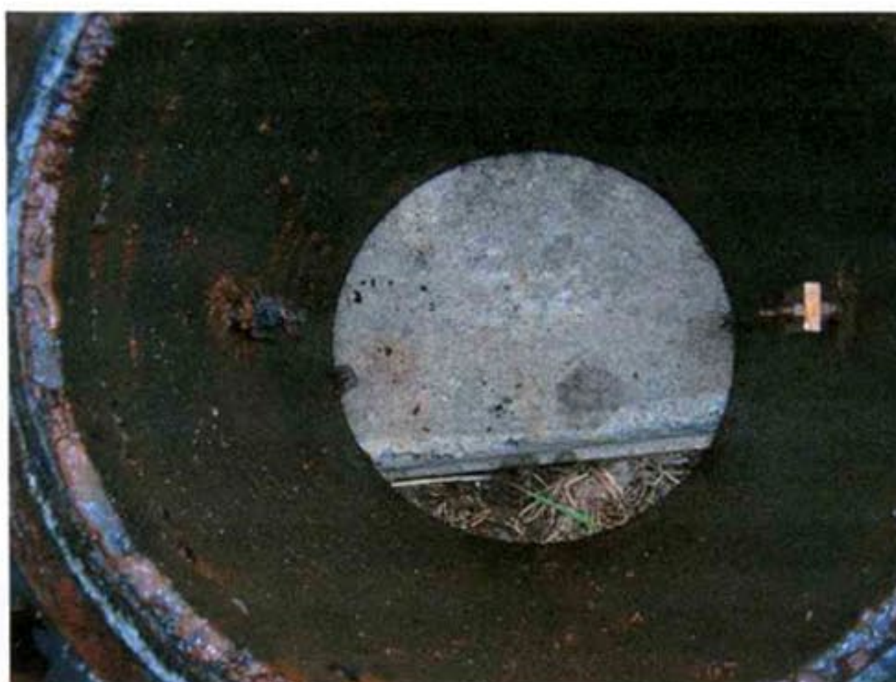
Fig.(11): Visual inspection of the Corrosion coupon ( to the left) and scale coupon (to the right)
